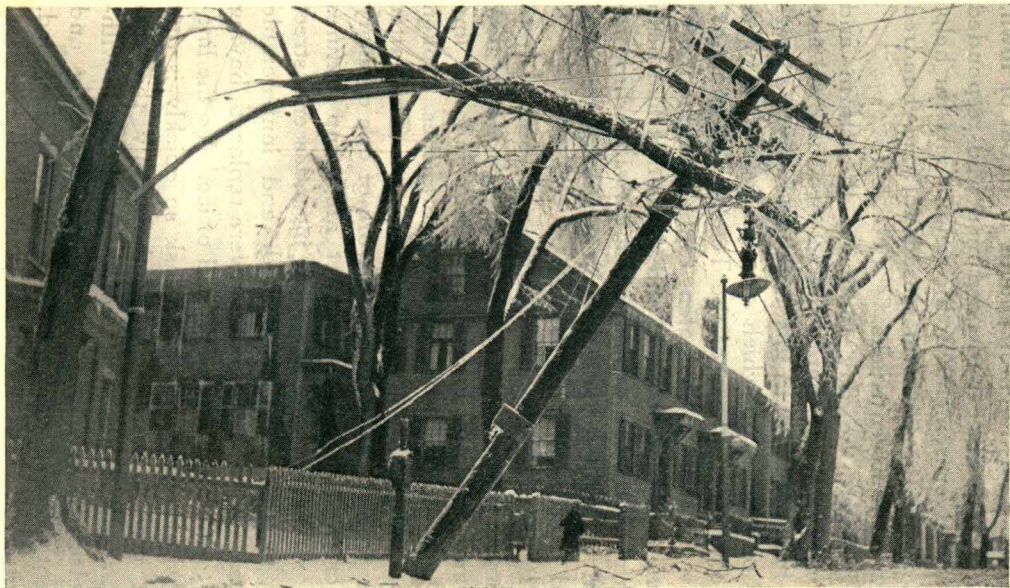
VIEW AT THE CORNER OF HIGH AND EAST MERRIMACK STREETS, LOWELL, SHOWING DAMAGE CAUSED BY FALLING LIMB.
